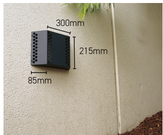
Flue cowl attached to external wall with Chateau installed into stud wall cavity
